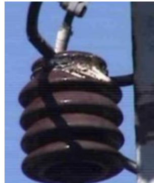
Fig. 9, 10. Corona discharge and its effects.
